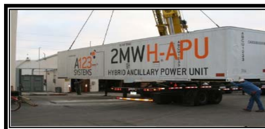
Figure K-2: Lithium-Ion Batteries
